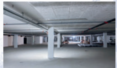
Parkhaus Grindelwald Terminal
